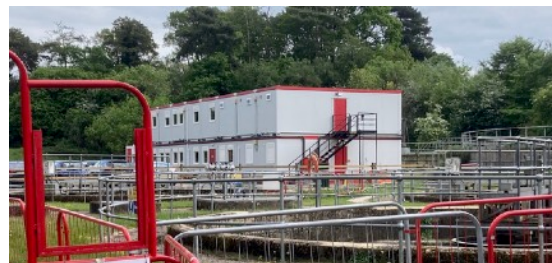
New Piggottshill Lane treatment works under development.
